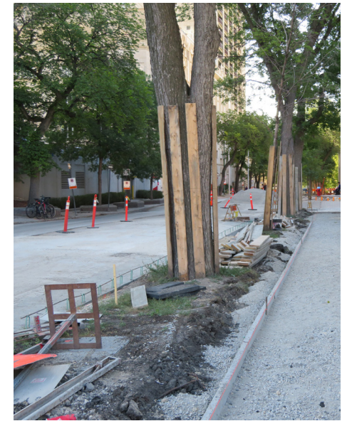
Tree damaged by poor pruning for new apartment building, not designed around the existing tree canopy (left). Inadequate tree protection led to blvd. damage during streetscape upgrades (right)
